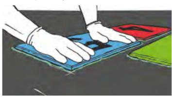
Apply the thick binder on outside edges of component to avoid edge separation from the rest of the EPDM on the top layer.
