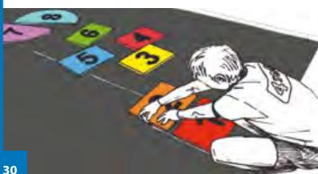
Mix properly two component glue. Use standard PU glue for artificial grass. Two component glue, use for bigger patterns or more graphics.
